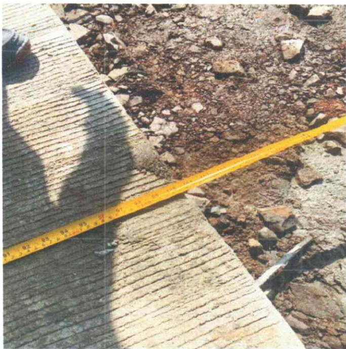
Concreting of Brgy Road (Phase II), Brgy. Guinbaoyan Sur- Tapae, Calbayog City
