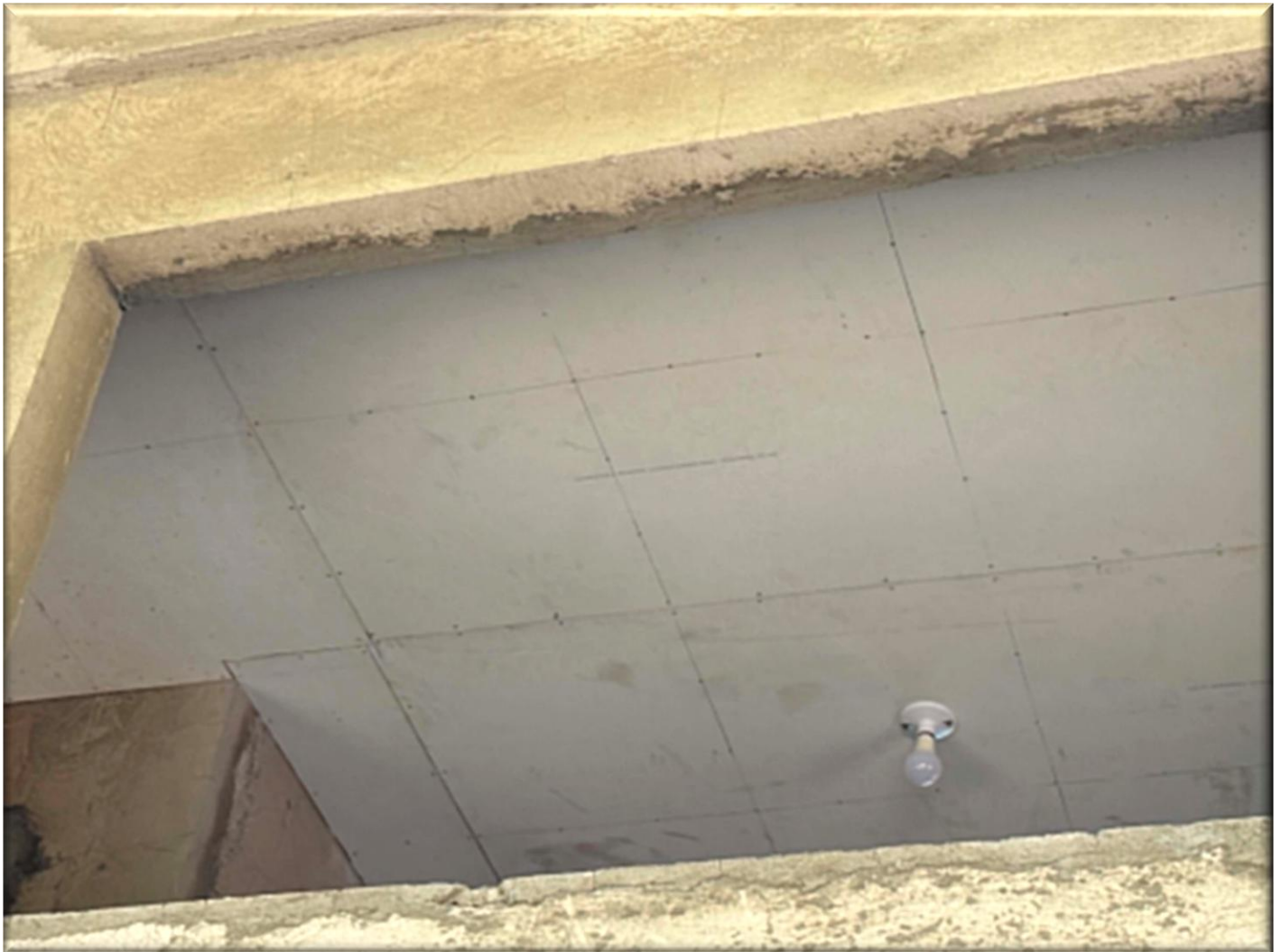
Ceiling of the 2 nd Floor
