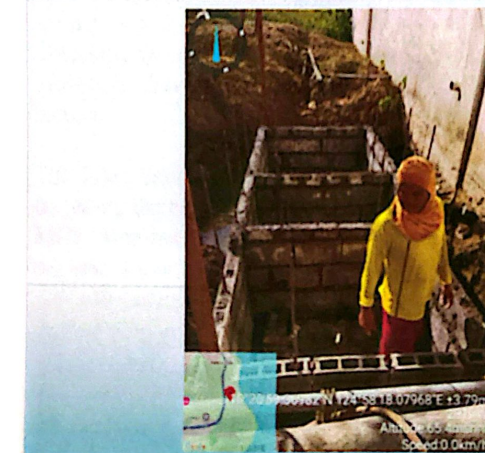
CONSTRUCTION OF SEPTIC TANK AT ISOLATION BLDG. Contractor: By Admin
