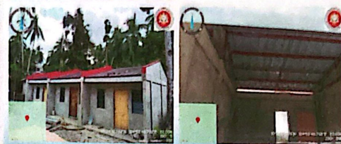
CONSTRUCTION OF SOCIALIZED HOUSING AT BRUY PONG-ON Contractor: Galat Construction Services
