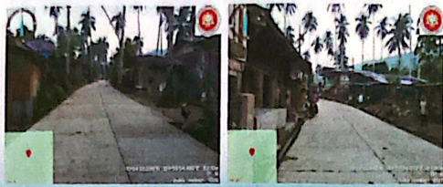
CONCRETING OF PURUK RAGA ROAD AT BRUY HILAAH Contractor: By Admin
