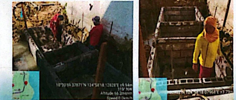
CONSTRUCTION OF SEPTIC TANK AT ISOLATION BLDG. Contractor: By Admin
