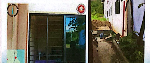
IMPROVEMENT OF EVACUATION CENTER Contractor: Galat Construction Services
