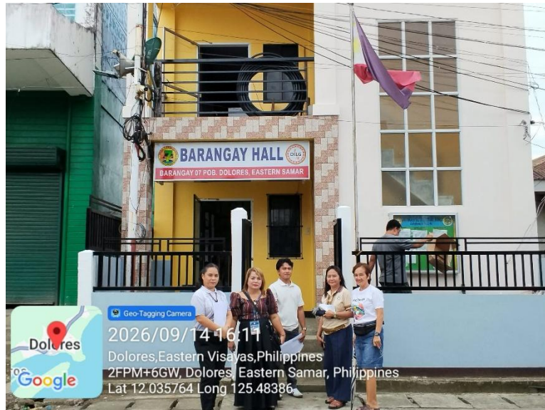
REHABILITATION OF MULTI-PURPOSE HALL (BRGY. HALL) BRGY. 07 DOLORES, EASTERN SAMAR
