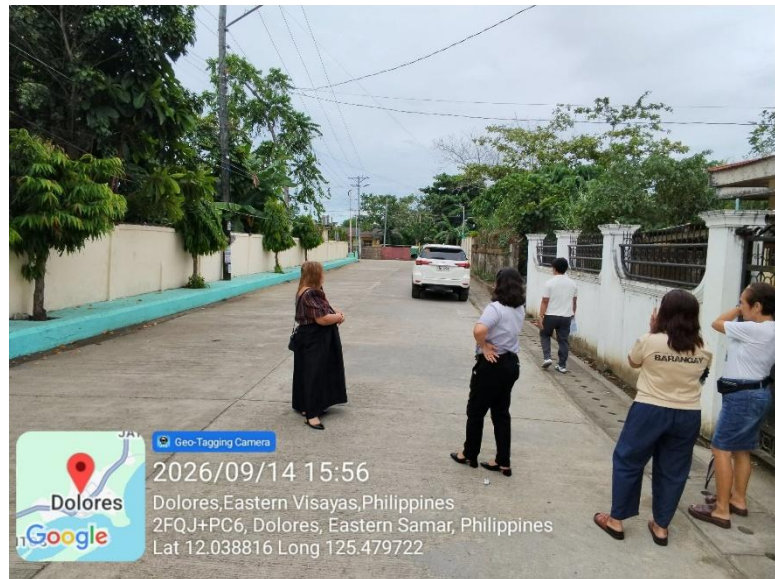
CONSTRUCTION OF DRAINAGE CANAL WITH CONCRETE COVER REYNALDO STREET, BRGY. 9 & 11, DOLORES EASTERN SAMAR
