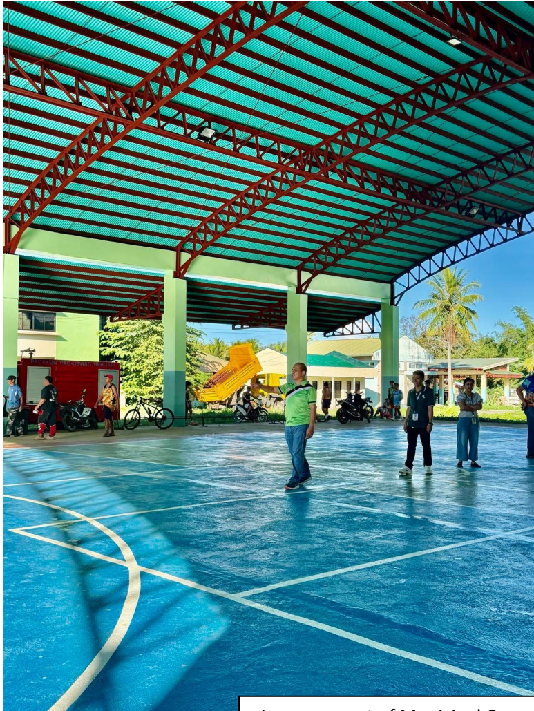
Improvement of Municipal Covered Court at Civic Center, Hernani, Eastern Samar
