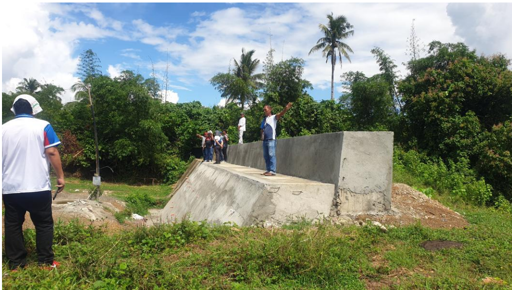
Construction of Slope Protection
