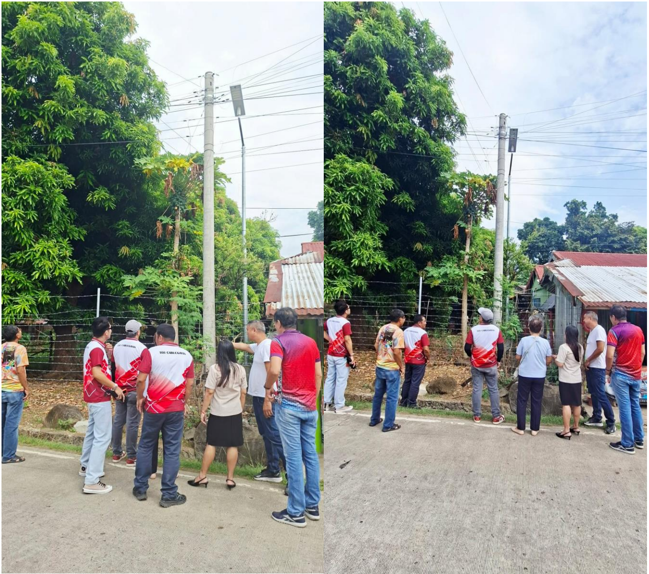
Solar streetlights with PLDT post obstructing the illumination of solar lights
