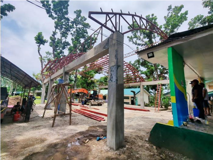
Name of Project: Construction of Mini Gym Location: San Agustin ES, Brgy. San Agustin Status: Ongoing
