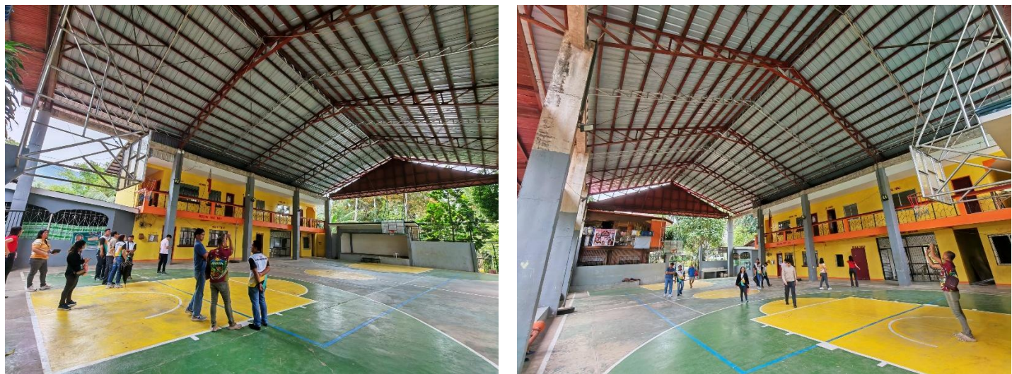
Name of Project: Construction/Improvement of Multi-Purpose Building Location: Brgy. Higulo-an Status: Completed
