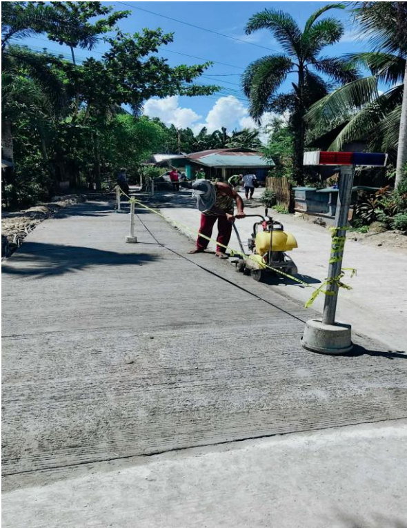
Road Concreting of Manlilisid to Cancayang, Javier, Leyte
