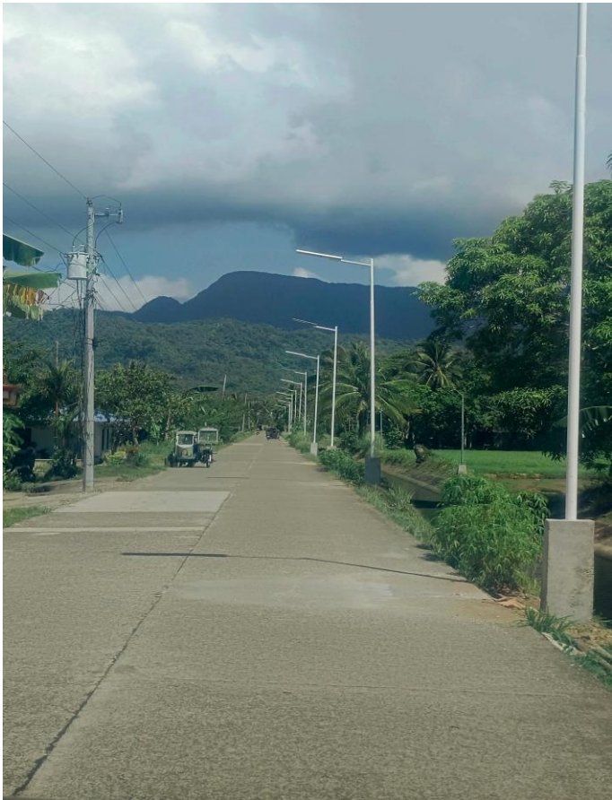
Solar Streetlights Installation
