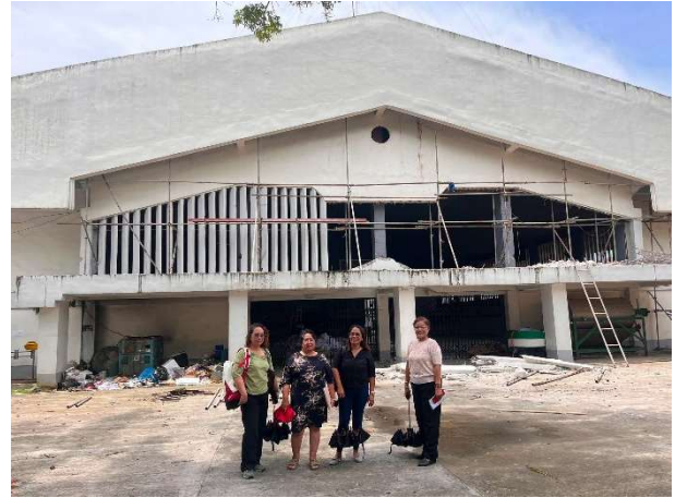
Rehabilitation of Multi-purpose Building at Brgy. Zone 3, Santa Fe, Leyte Project Cost: 50,000,000.00
