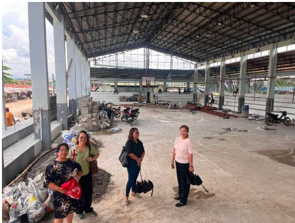
Upgrading and/or Improvement of Municipal New Public Market Covered Court – Canopy and Bleacher (Phase 2), Brgy. Zone 2, Santa Fe, Leyte Project Cost: 4,325,000.00
