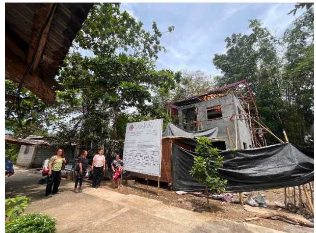
Construction of 2-storey Multi-purpose Building, Brgy. Zone 4, Santa Fe, Leyte Project Cost: 2,510,000.00
