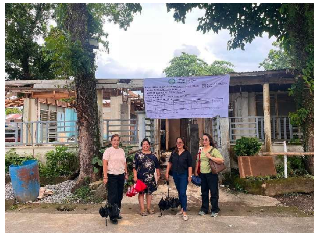
Renovation, Repair and/or Improvement of Old RHU Building, Brgy. Zone 2, Santa Fe, Leyte Project Cost: 1,500,000.00
