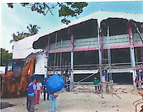
Rehabilitation of Multi-purpose Building at Brgy. Zone 3, Santa Fe, Leyte Project Cost: 50,000,000.00
