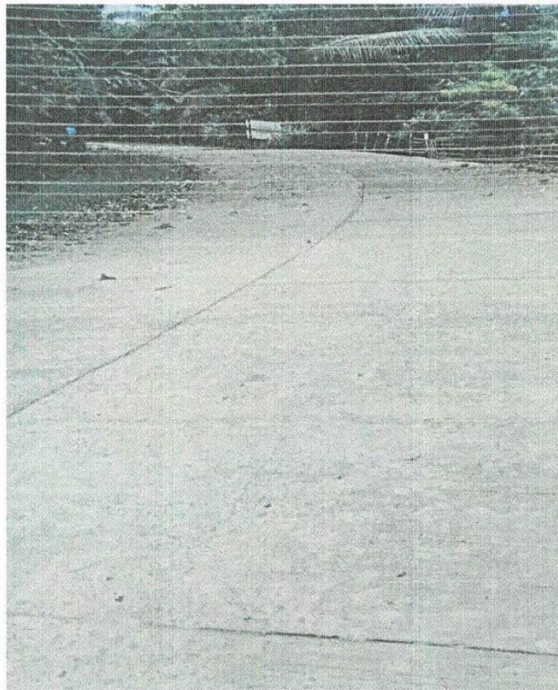
Project Title: Road Concreting Location: Proper, Brgy. Butason 1, Tabango, Leyte
