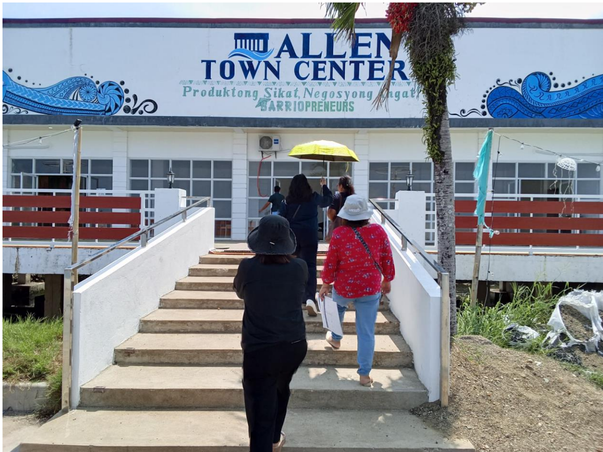
Construction of Multi-Purpose Bldg. at Kinabranan Z-I
