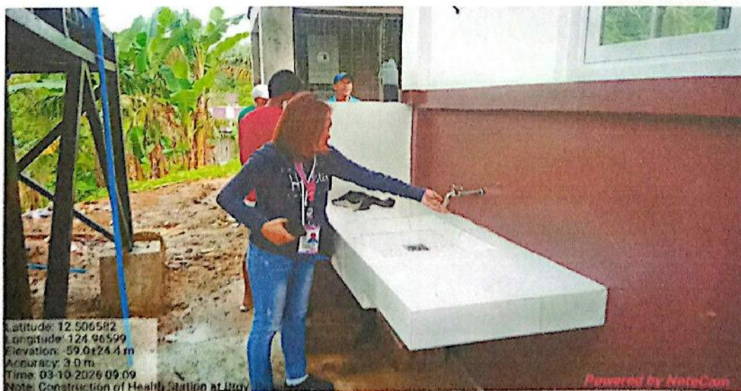
March 10, 2026 – Construction of Health Station at Brgy. Palmera, Laoang, Northern Samar
