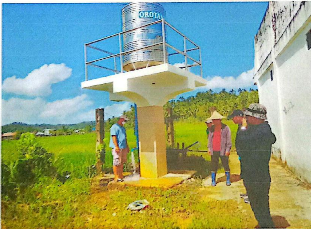
January 22, 2026 – CONSTRUCTION OF MODEL FARM WITH GREEN HOUSE AND WATER SYSTEM AT CANGCAHIPOS DEMO FARM, BRGY. CANGCAHIPOS, LAOANG, NORTHERN SAMAR
