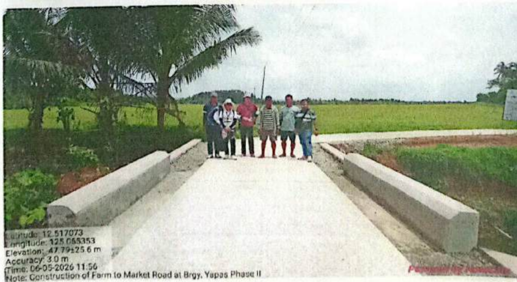
June 5, 2026 – Concreting of Farm to Market Road at Brgy. Yapas Phase II, Laoang, Northern Samar
