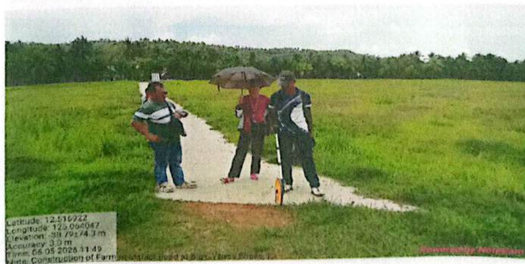
June 5, 2026 – Concreting of Farm to Market Road at Brgy. Yapas Phase II, Laoang, Northern Samar
