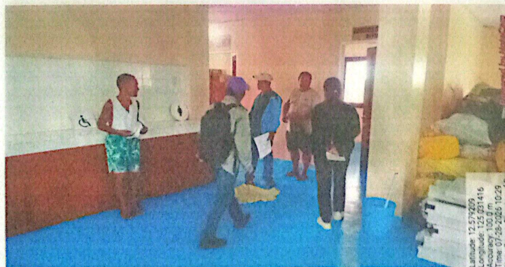
JULY 28, 2026 – REPAIR FLOORING OF BRGY. AGUADAHAN COMMUNITY EVACUATION CENTER
