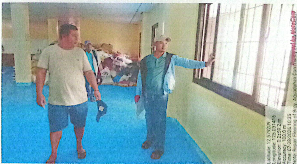
JULY 28, 2026 – REPAIR FLOORING OF BRGY. AGUADAHAN COMMUNITY EVACUATION CENTER
