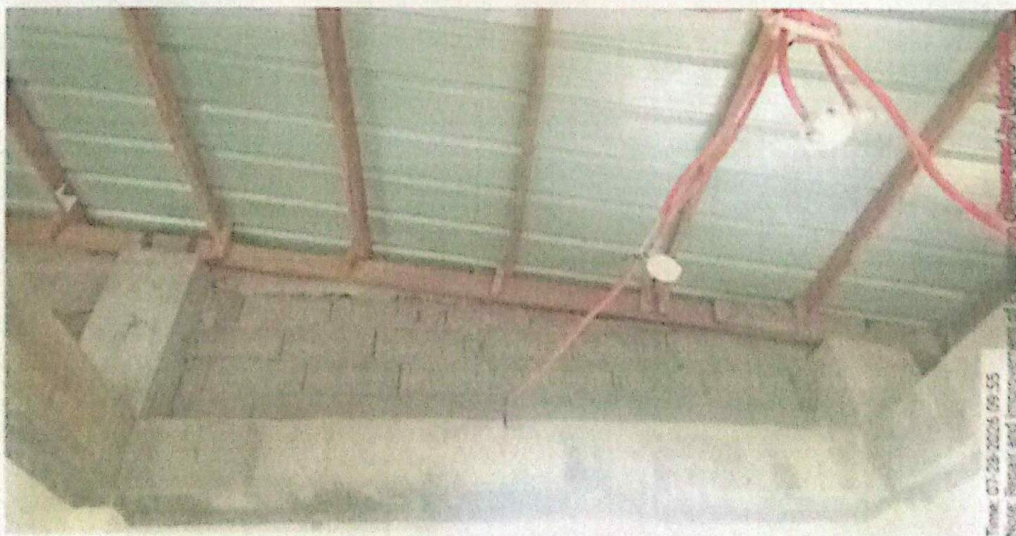
JULY 28, 2026 – REPAIR AND IMPROVEMENT OF EVACUATION CENTER IN BRGY. LANGOB
