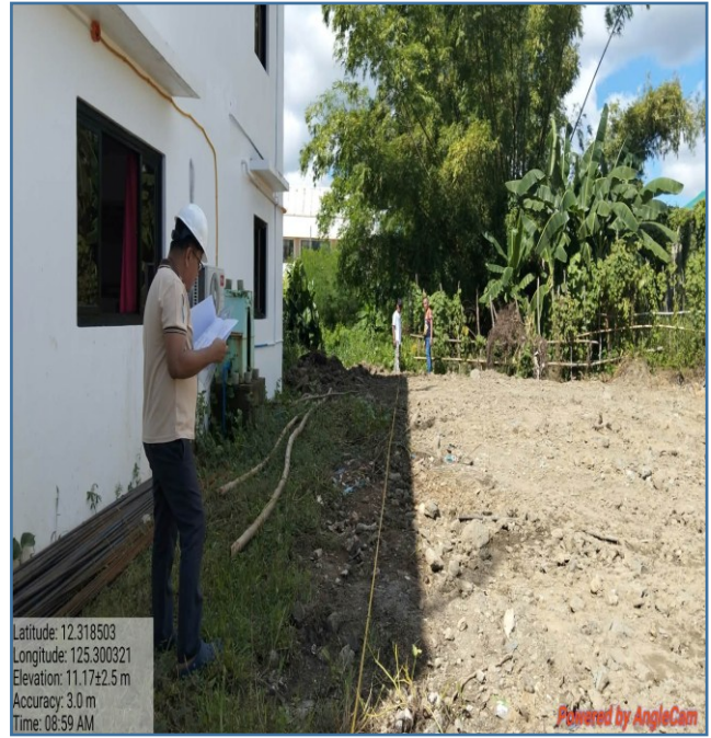
Construction of Multi Purpose Building (Motor Pool) at Lapinig Del Norte
